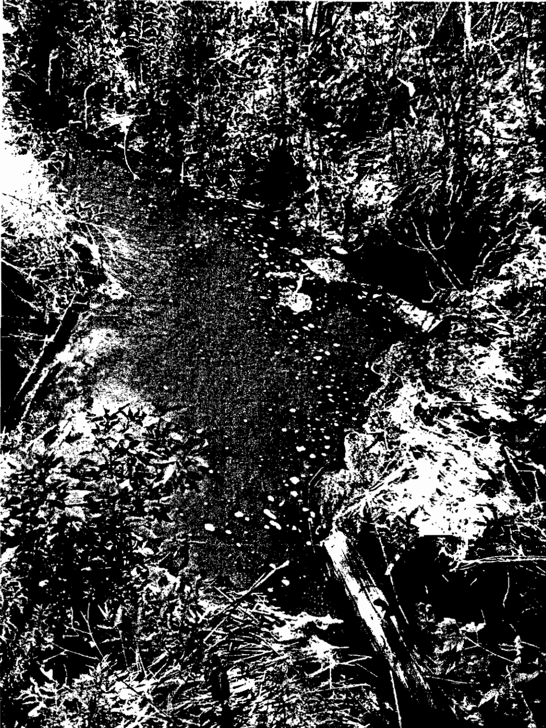
Photograph 5: Same location as photograph 4, looking east. Photograph shows flowing water in the Southside Canal. The water was flowing from the east to the west or from the top left corner to the lower right corner in the photograph. The buildup of branches and a large log caused the pooling of water both above and below the debris.
